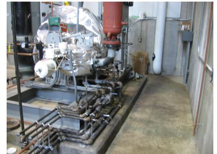
A small induction unit is used in lieu of an energy wasting pressure reducing station helping reduce a college's total energy costs.
